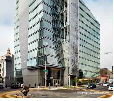
The San Francisco Public Utilities Commission Headquarters features *Solarban*® 70 glass over *Starphire*® glass by Vitro Architectural Glass (formerly PPG glass). As a result of natural daylight harvesting made possible by the high-performing glass, the building uses less energy for interior illuminations than a typical office building.
